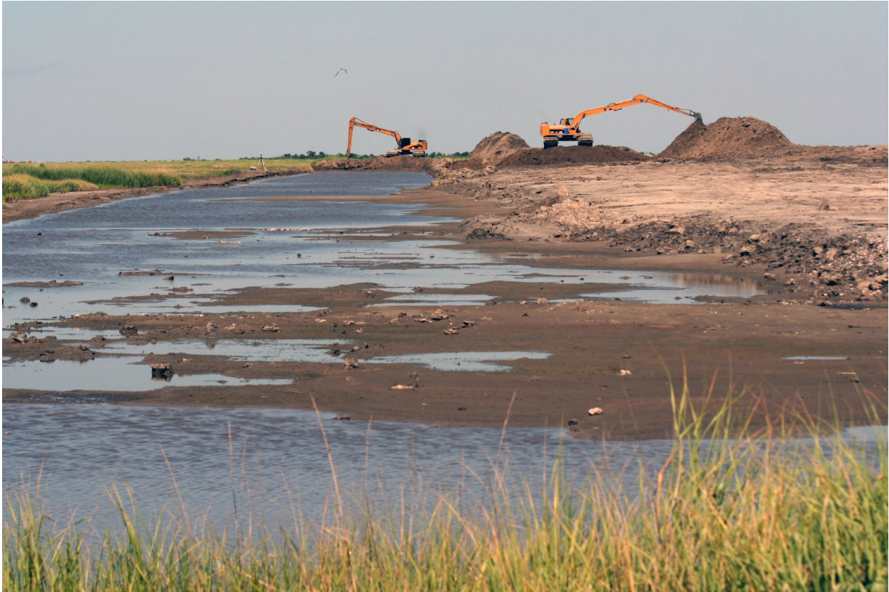
Figure 6 Excavators digging down fill to marsh elevation and stacking the material to build up the elevation of the ridge. South marsh apron of Far Ridge, May 29, 2008, looking west.
