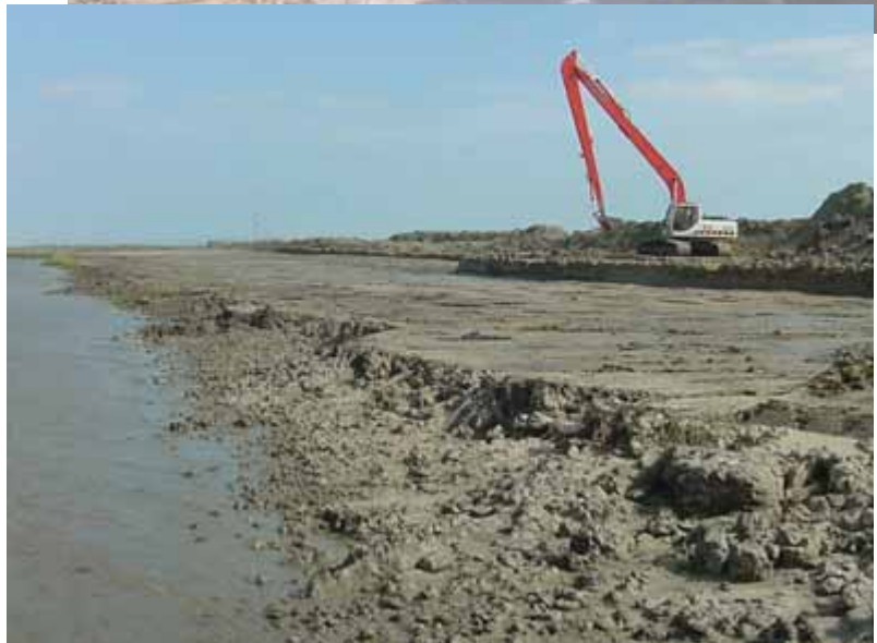
A bucket dredge shapes newly pumped material on the Port Fourchon Maritime Ridge.
