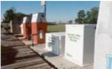
A typical pumpout system, courtesy of LDWF Clean Vessel Act Program.
