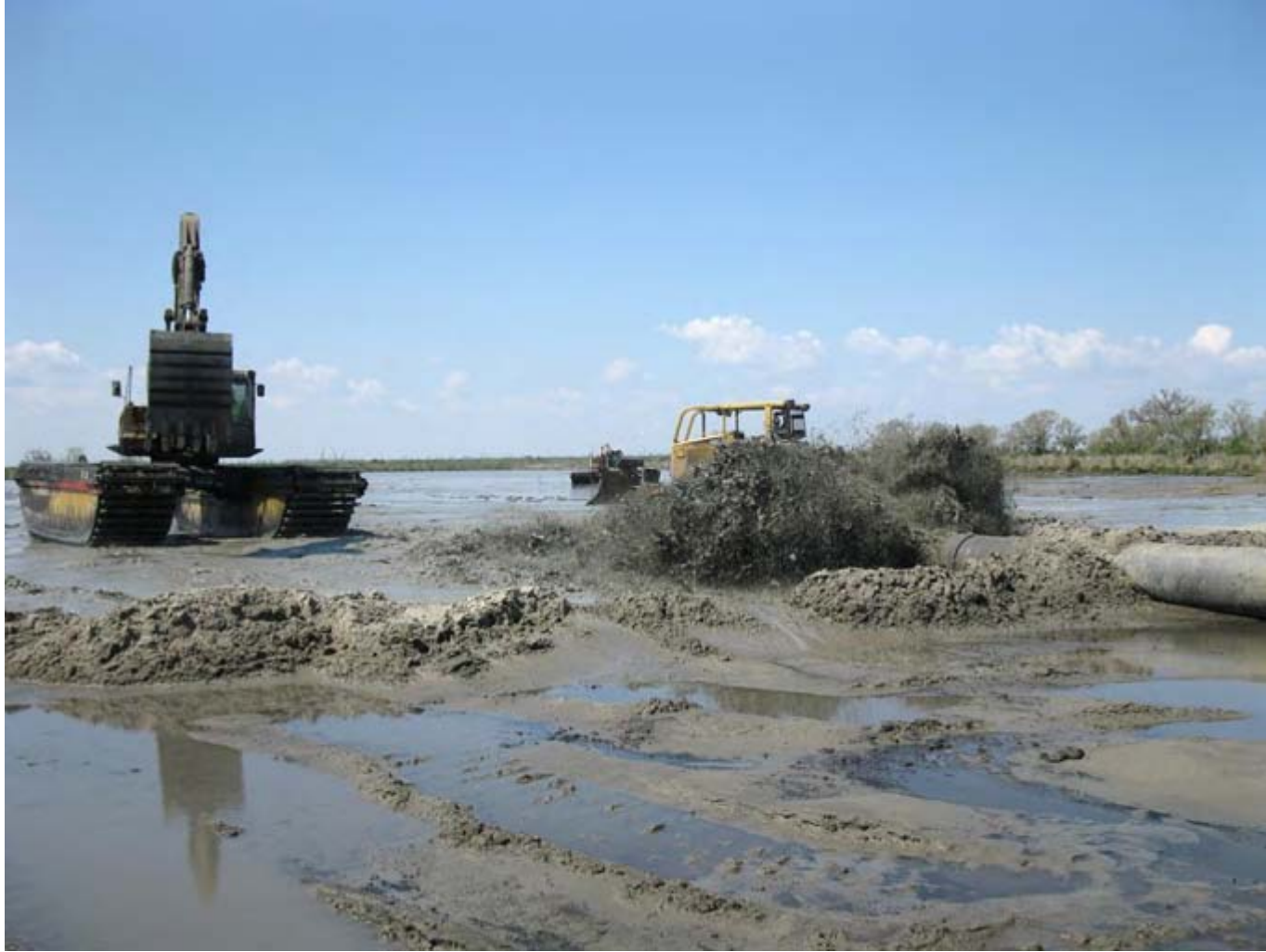
Slurry Pipe Discharge in Marsh Creation Area
