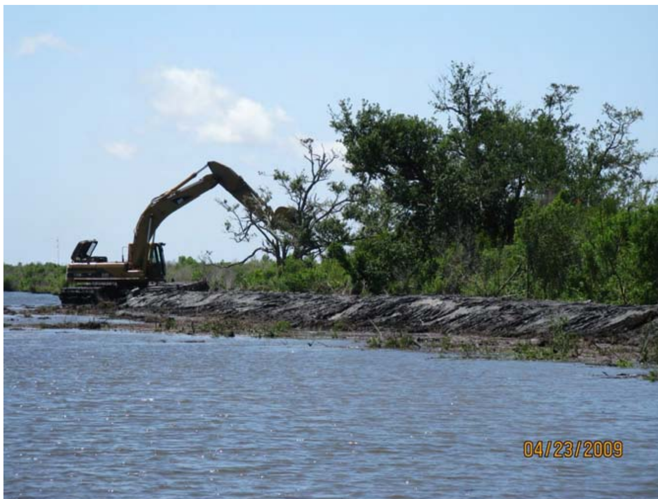
Building Enhanced Spoil Bank
