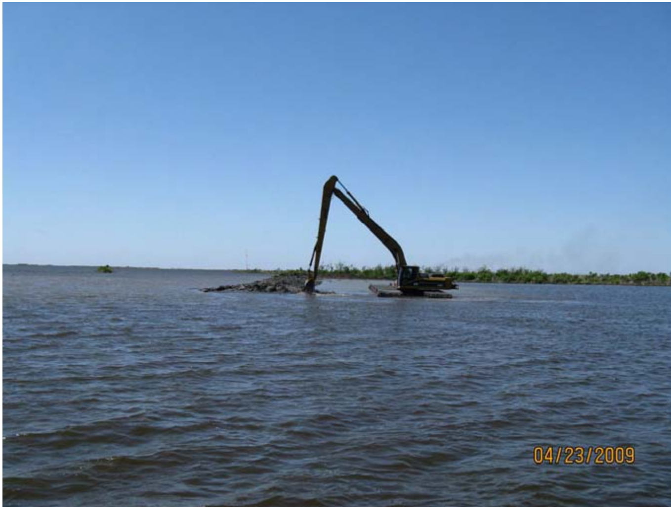
Building Earthen Containment Dike in Open Water
