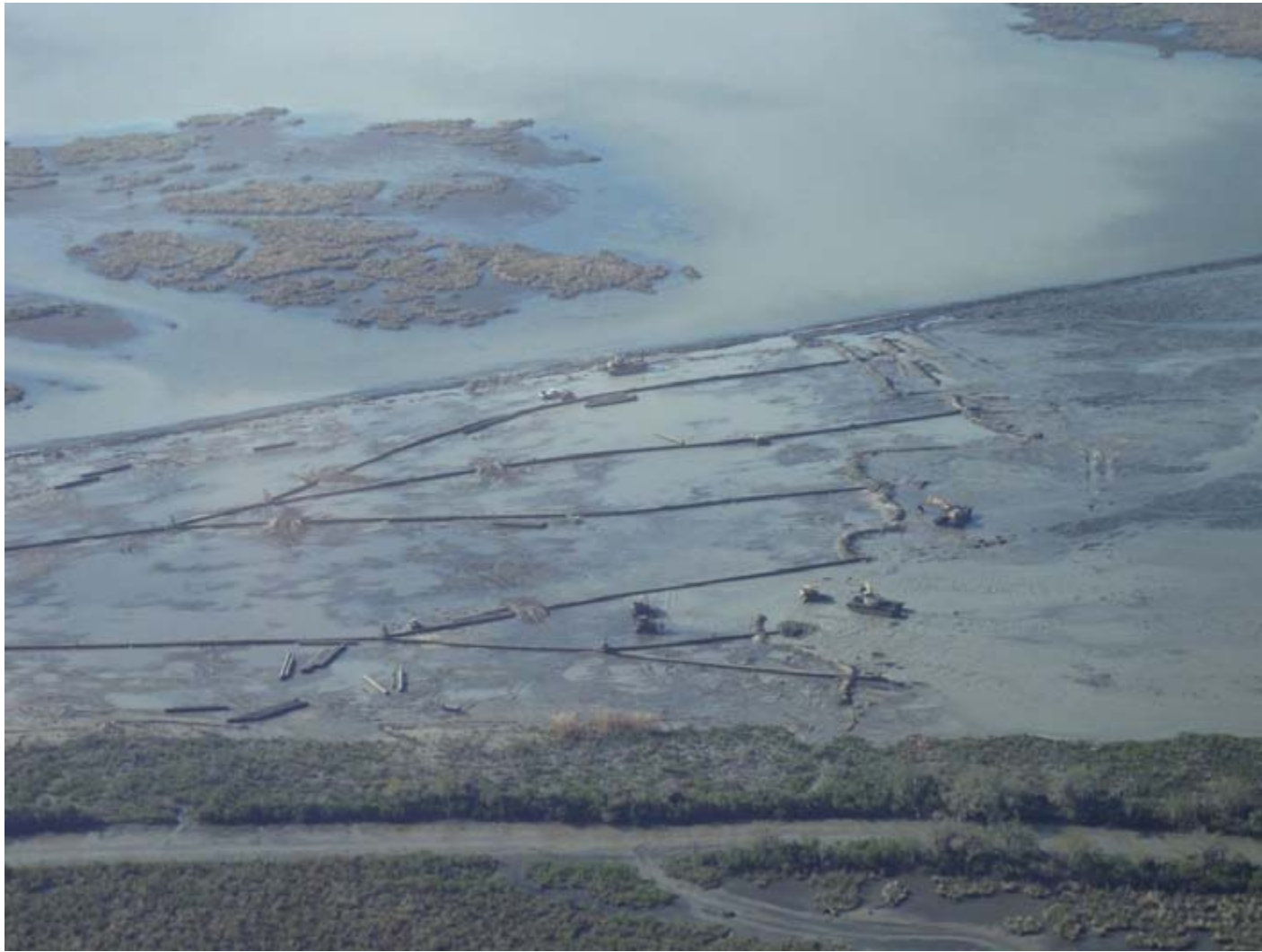
Multiple Distribution Lines Helped Speed Filling of Increment 2
