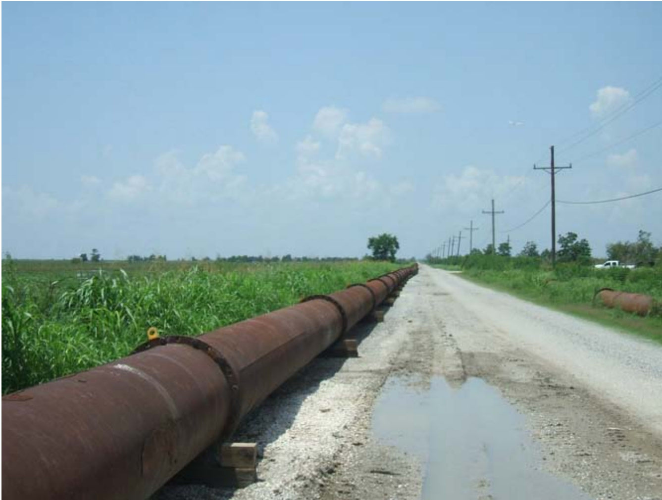
9,000' Flanged Joint Pipe
