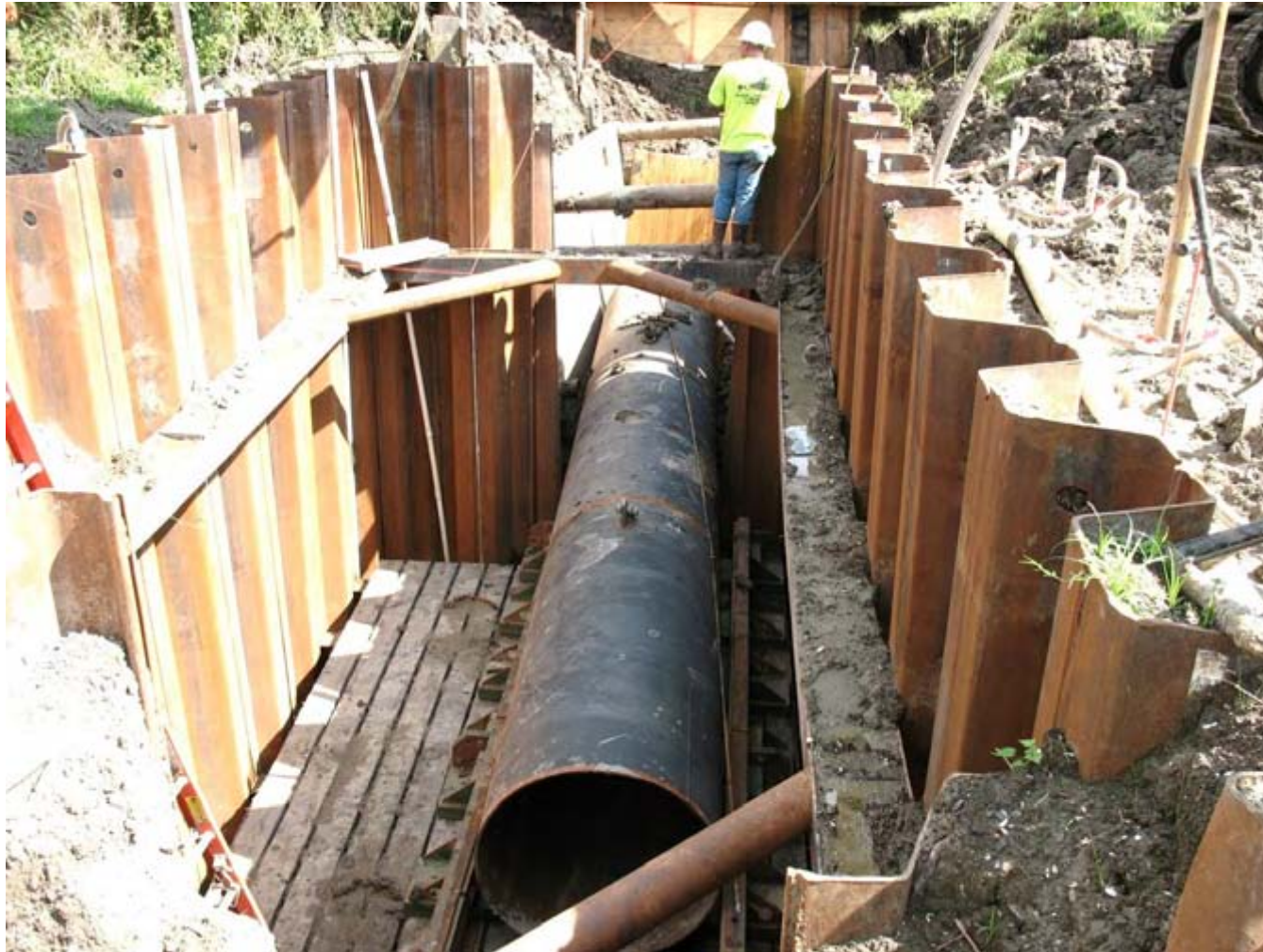
48" dia. Casing in Cofferdam
