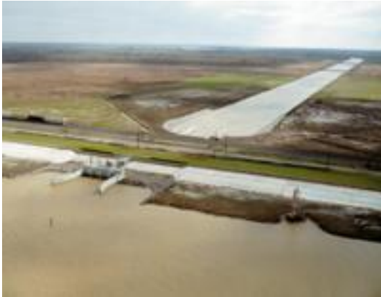
Davis Pond Diversion Structure
