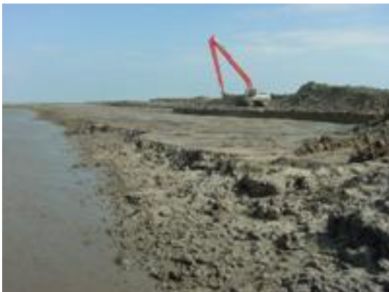
Excavator on the Maritime Forest Ridge
